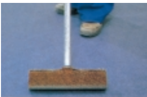
Rubbing down the sheets with a rubbing iron, a device covered with needle felt...
