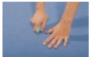
A useful tip if the trapped air cannot be forced out laterally: make a small hole with the point of a blade in a dark section of the pattern, press out the air and once again firmly rub down the covering at this point.
