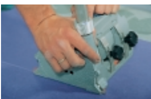
Milling out the joint.
