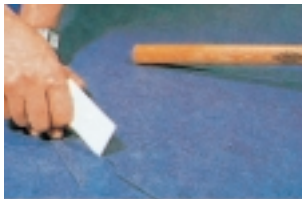
The seam should never fit too tightly. There should be a space of approx. 0.5 mm between adjoining edges when sealing.
