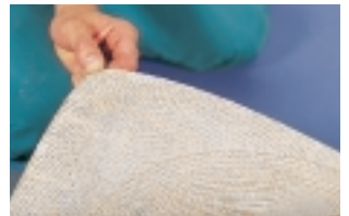
Adhesive must be applied in such a way that the strips of adhesive cover the entire backing of the floor covering.
