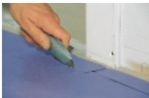
The covering is cut along the scored contours.
