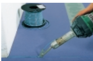
Sealing with a manual welder.
