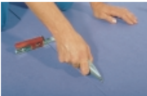
Trimming the top edge with a hooked knife.
